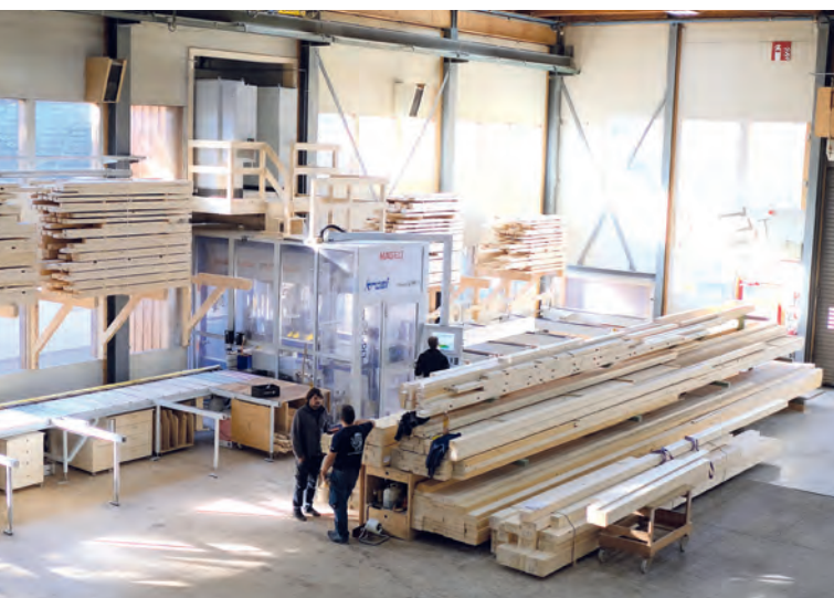
Space-saving: The Krüsi MC 15 was installed "in the wall" and the control cabinets above the machine.
