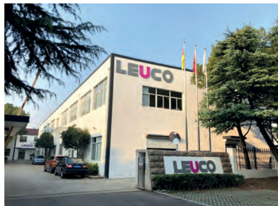
| LEUCO China Headquarters in Taicang
